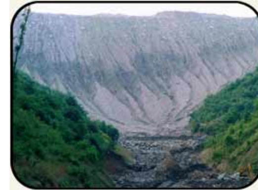
Appalachian stream fill. Photo by Bob Gates from OVEC.
